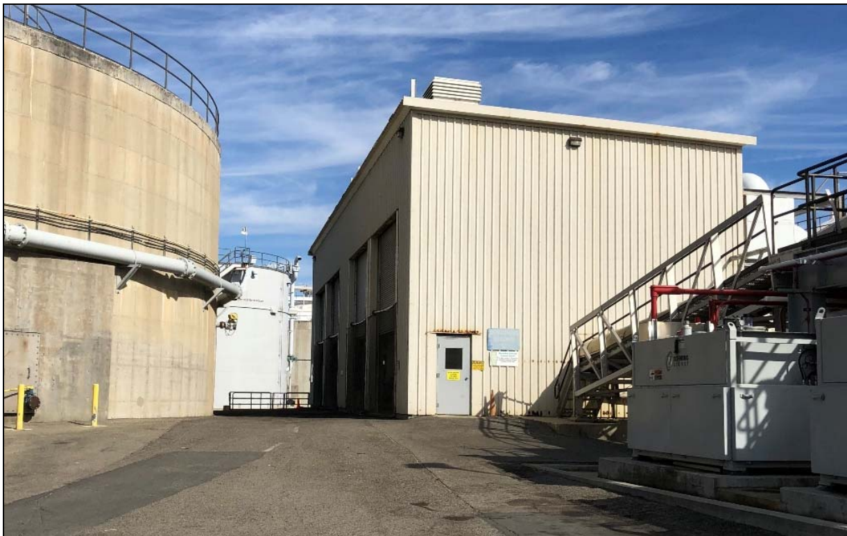
Dewatering Building C (view facing north) (ESA, 2018)
