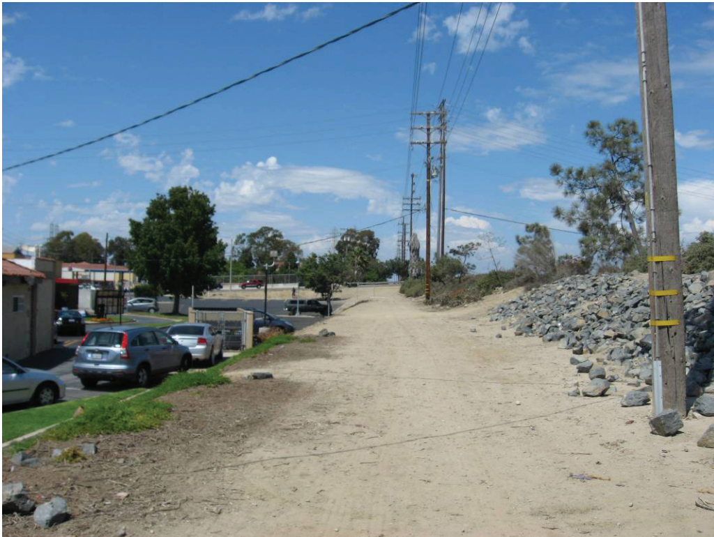
Photo 7: Second pipeline entry location along the OCSD easement corridor.
