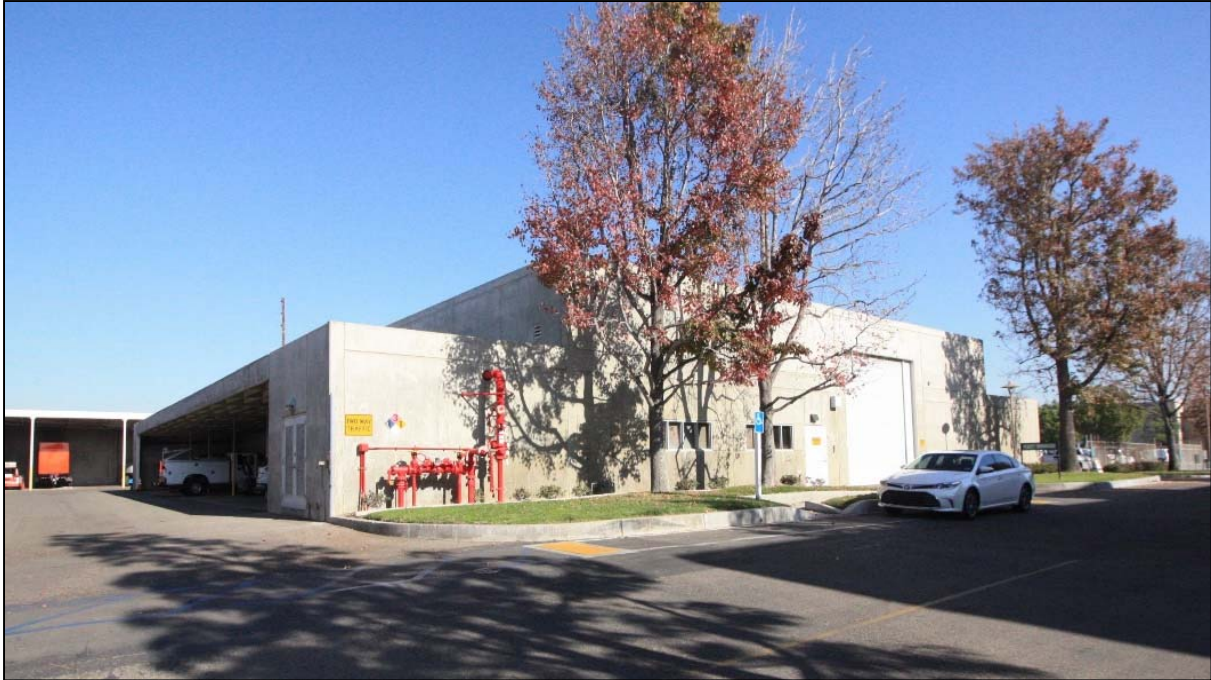
Primary elevation of the Fleet Services building, view facing north (ESA, 2018)
