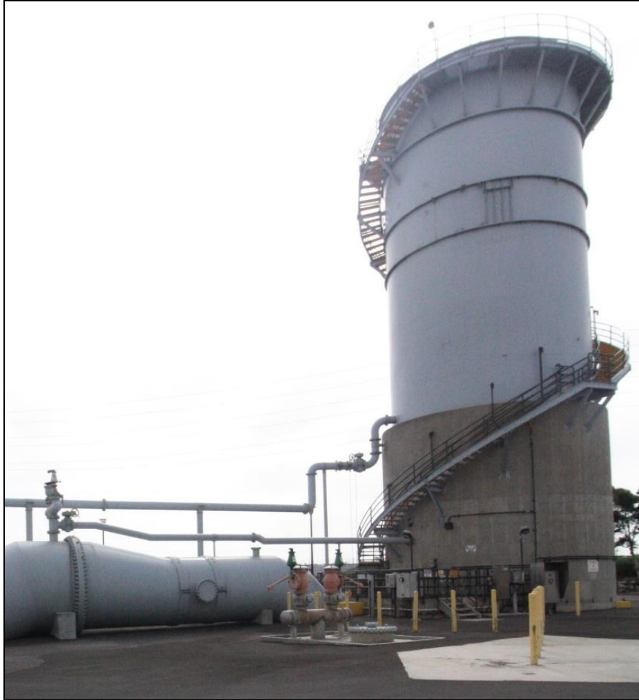
Figure 15 View of Surge Tower No. 2 and adjacent outfall pipe (view facing east)
