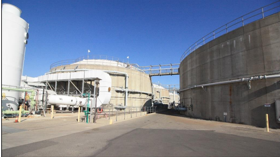
Orange County Sanitation District Plant No. 1 – 150626.00
