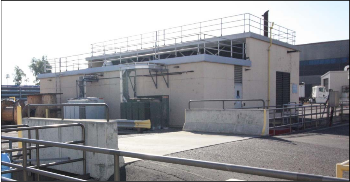
Power Building 2, view facing south (ESA, 2018)
