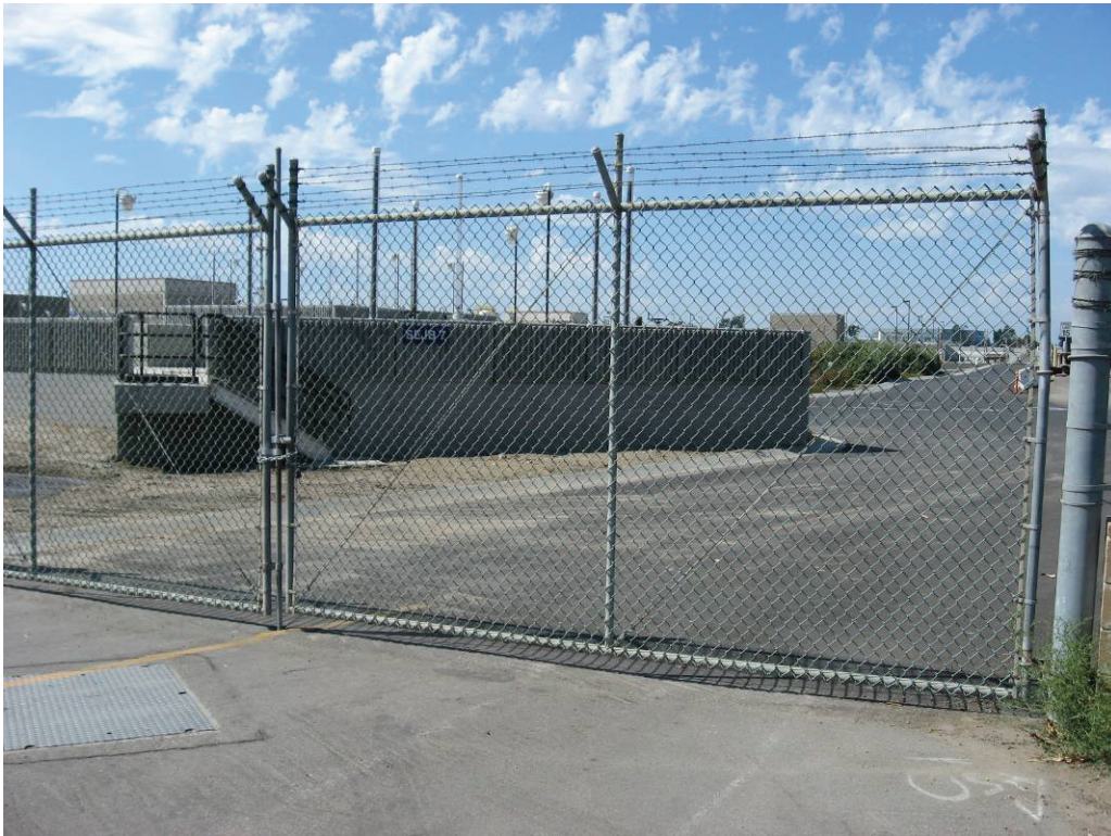
Photo 15: OCSD Pipe Connection to existing facilities. Note the area is paved and previously disturbed during construction of the facility.
