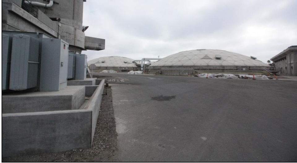
Orange County Sanitation District Plant No. 2 – 150626.00
