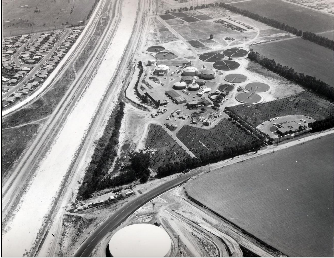
Orange County Sanitation District Plant No. 1 – 150626.00
