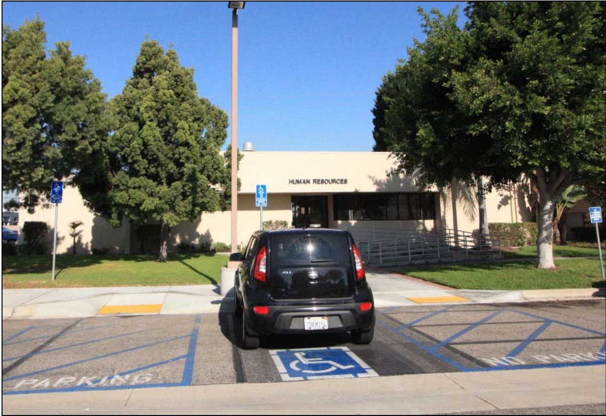
Human Resources building primary elevation, view facing north (ESA, 2018)
