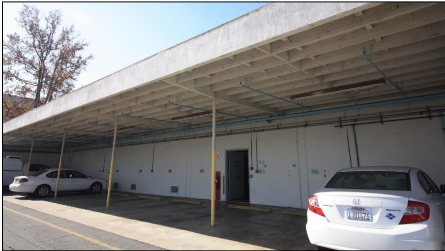
Orange County Sanitation District Plant No. 1 – 150626.00
