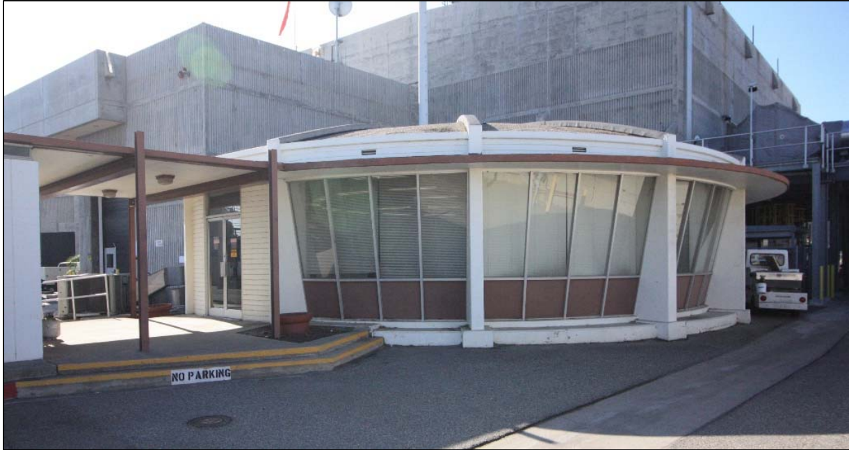
Old Operations Control Center, view facing west (ESA, 2018)
