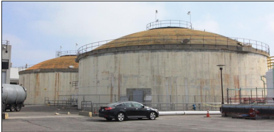
Orange County Sanitation District Plant No. 2 – 150626.00
