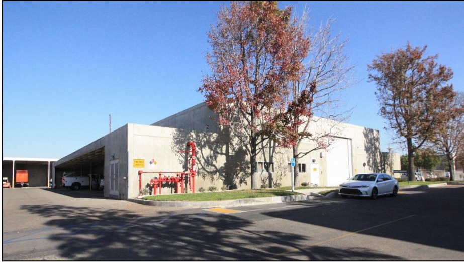
Orange County Sanitation District Plant No. 1 – 150626.00
