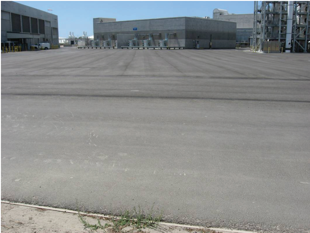
Photo 3: Pump Station and Pipe Connection; facing west.
