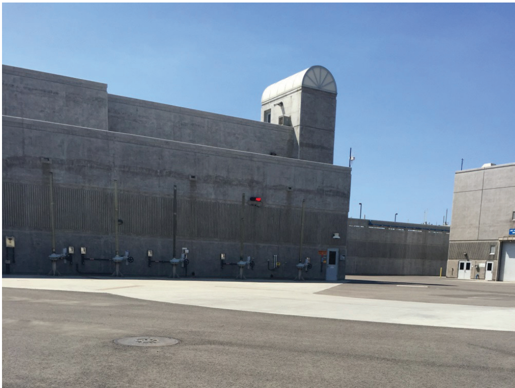
Photo 4: Headgates and Bypass Pipeline location.
