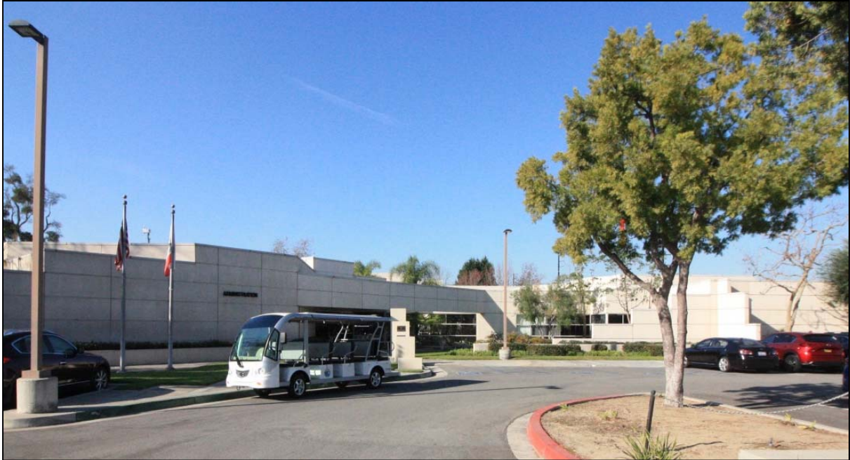
Administration Building's primary elevation, view facing west (ESA, 2018)
