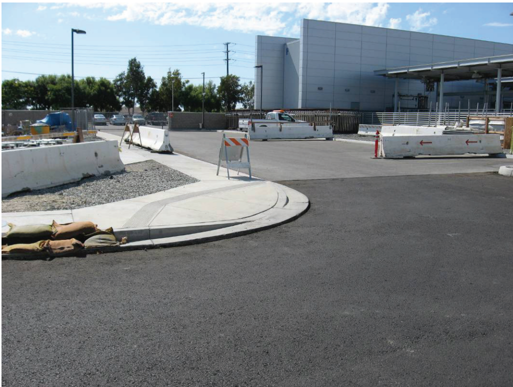
Photo 16: MF Building Expansion location; facing west.
