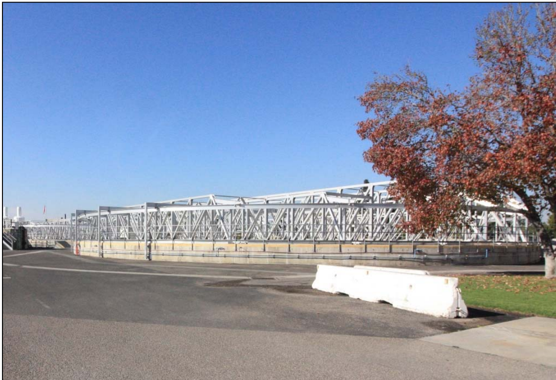
Primary Clarifiers 3 and 4, view facing west (ESA, 2018)
